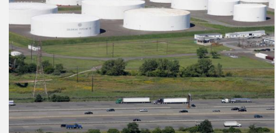
Ransomware Attack Shuts Down A Top U.S. Gasoline Pipeline
